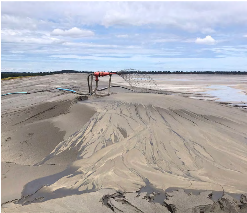
Pictured above: TSF cyclones at Kansanshi, Zambia
