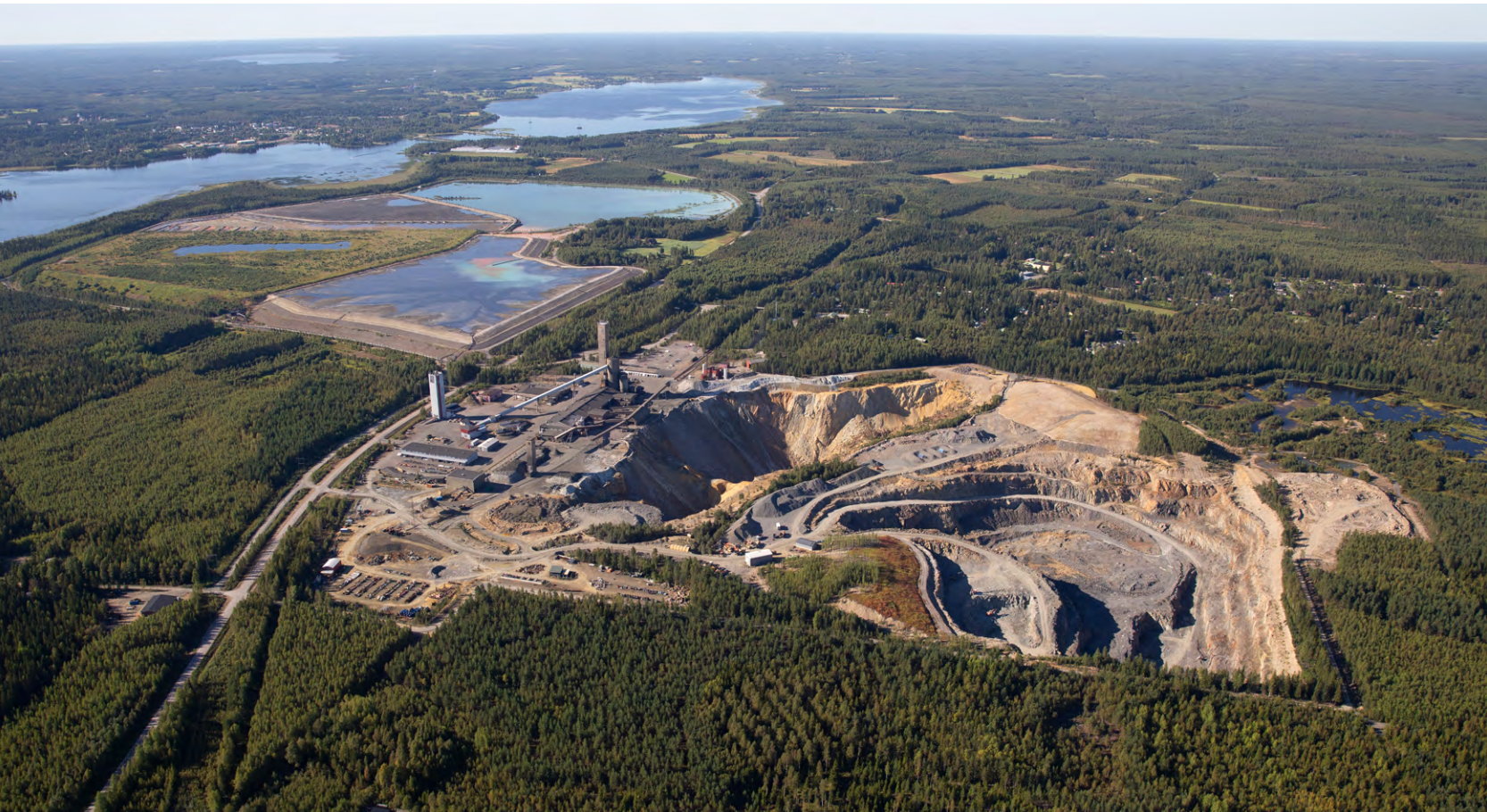
Pictured left: TSF at Pyhäsalmi, Finland
