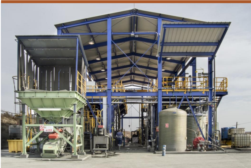
Las Cruces Poly Metallurgical Refinery Pilot Plant
