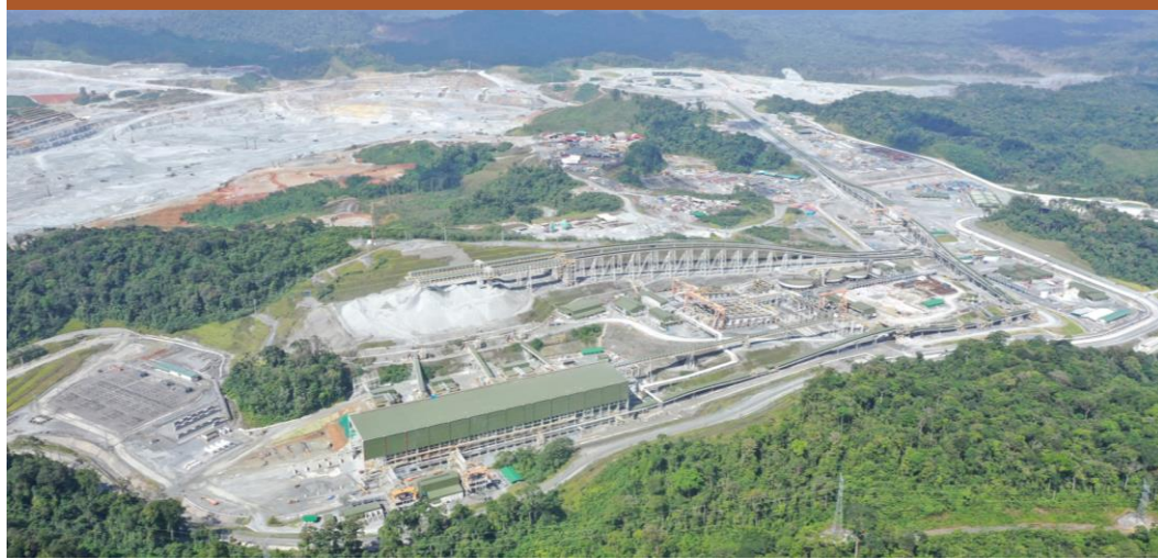
Process Plant and Pit
