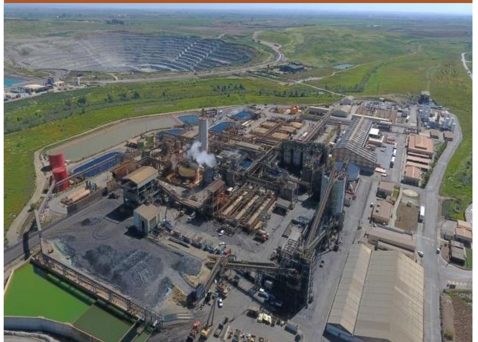
Las Cruces Plant and Open Pit
