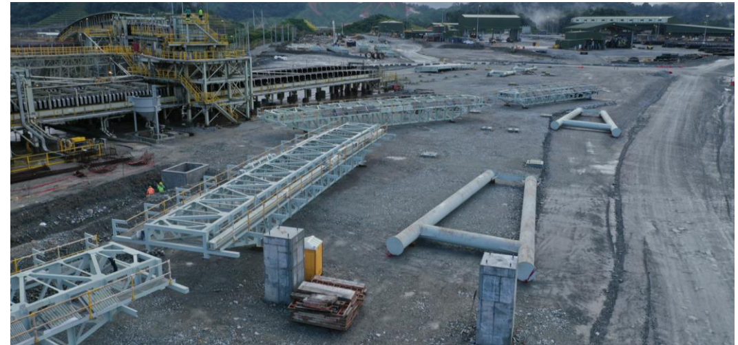
Screening Conveyors Progress
