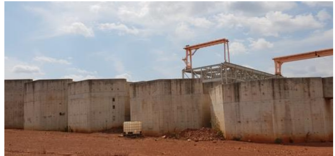
S3 Rougher Flotation Cell Pedestals
