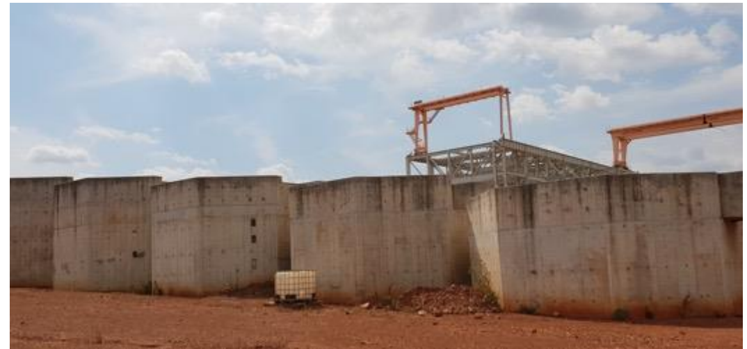
S3 Rougher Flotation Cell Pedestals
