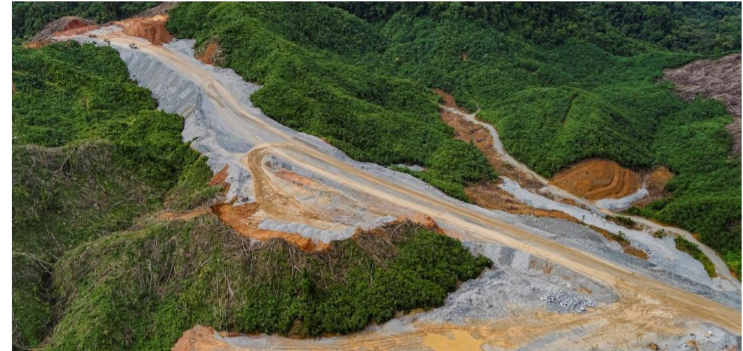
Colina Pit Access Road at Cobre Panama
