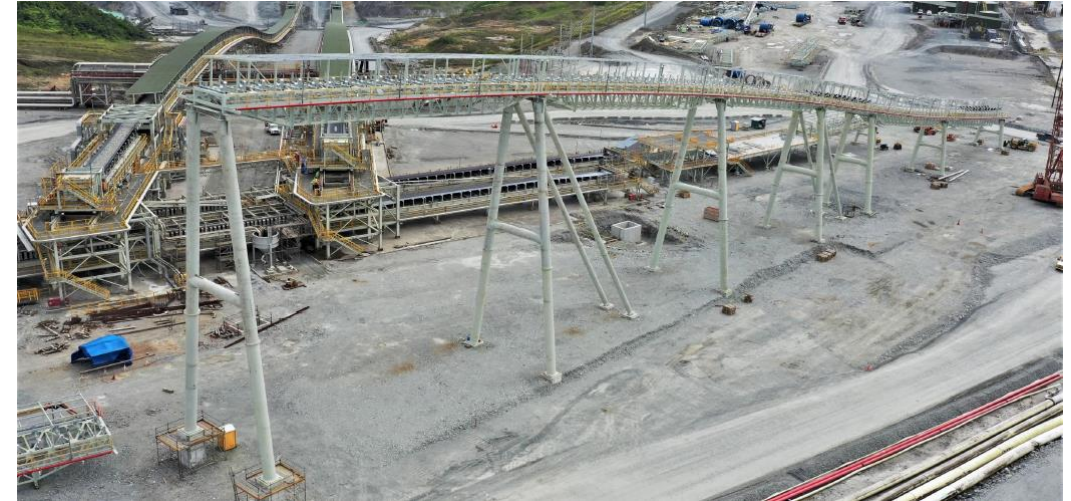
Screening Conveyors Progress
