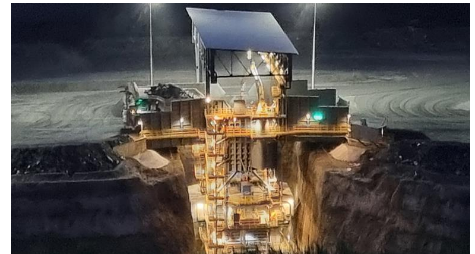
Sentinel Fourth In-Pit Crusher
