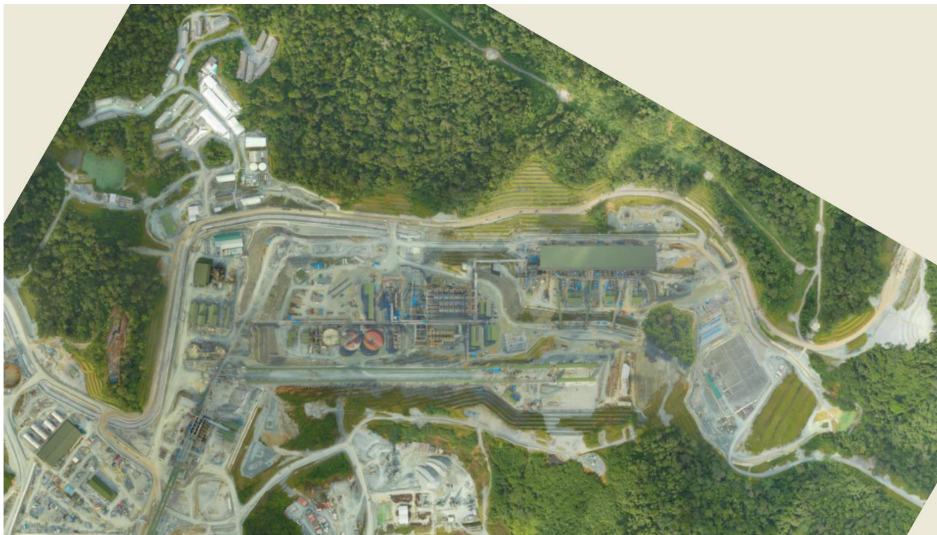
Figure 18-3 Photograph of as-built plant, December 2018
