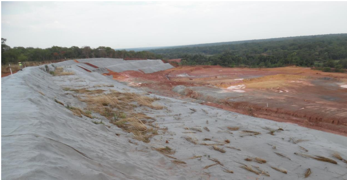
Figure 16-32 View looking north west over the Enterprise starter pit, October 2019
