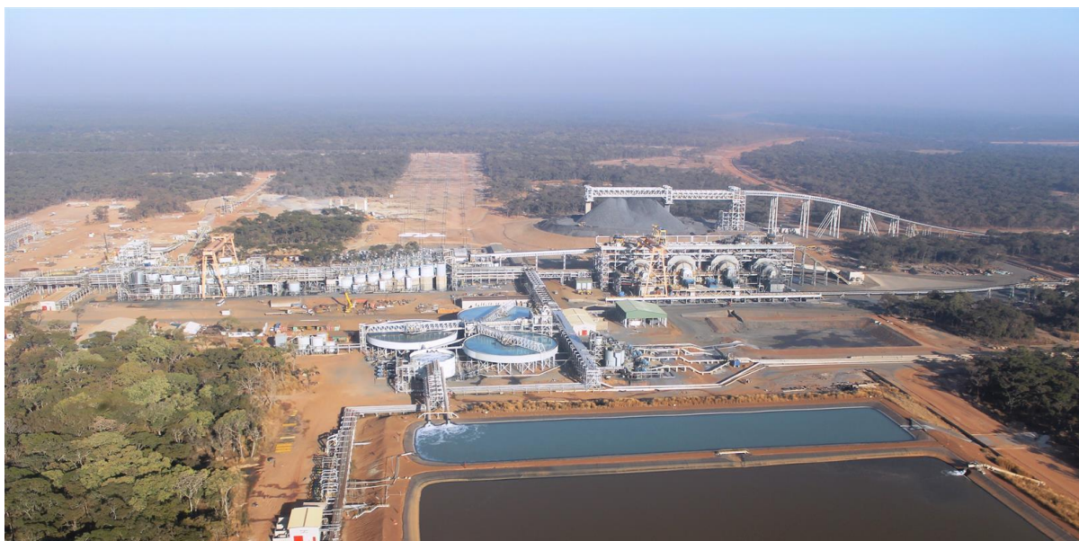
Figure 17-1 View looking west over the processing plant
