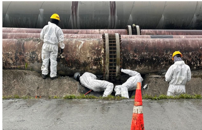
Tailings line – Inspection and bolt replacement
