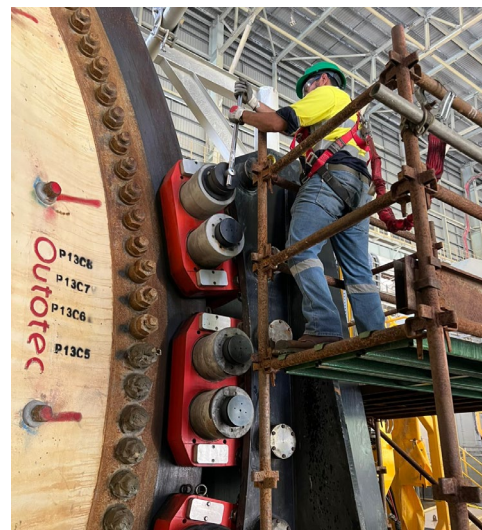
SAG Mill 4 brake maintenance
