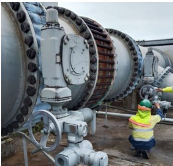
Process – Water pump valve change
