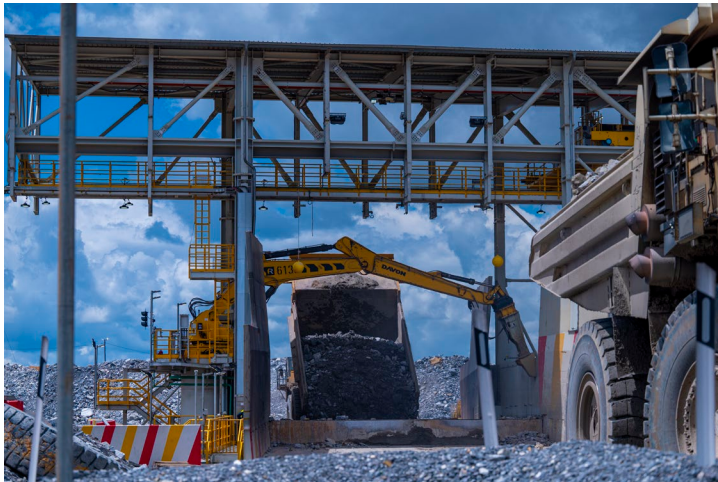
Delivering Ore to Crusher
